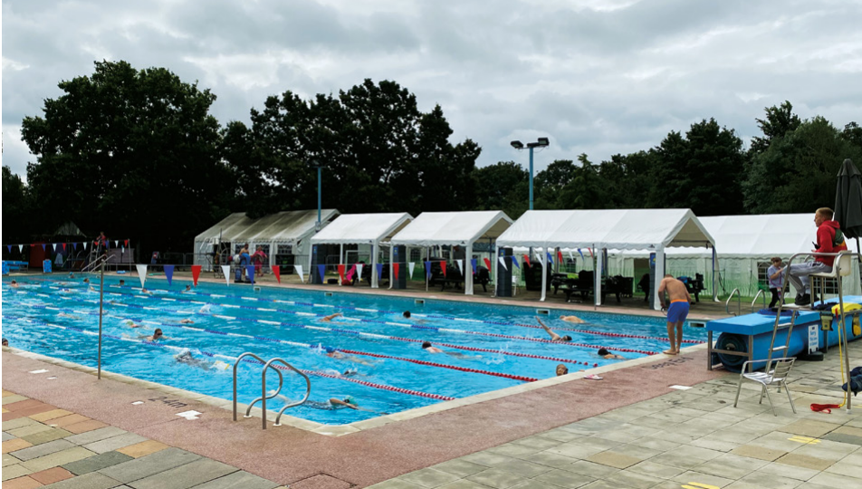
Inside-out at Hampton Pool
